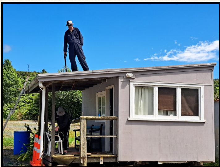
Trevor Townsend water blasting his hut roof in preparation for painting (Richard.E)
